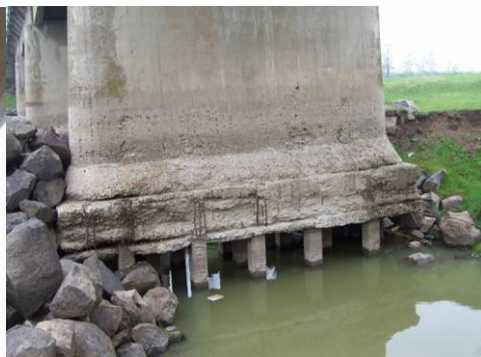
Figure 3. Pier founded on piles
