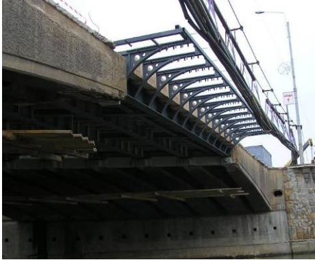
Figure 11. The new steel footway cantilivers
