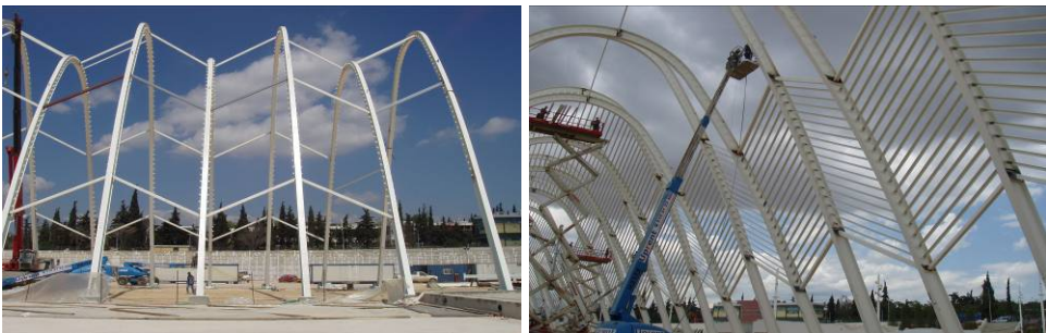
Figures 26 and 27. The AGORA during the erection
