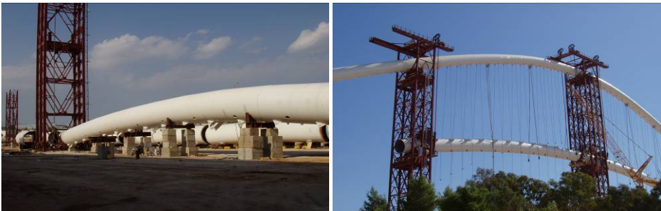
Figures 9 and 10. The arches during preparation and their erection
