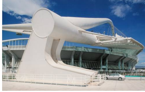
Figure 14. One of the four supports of the roof
