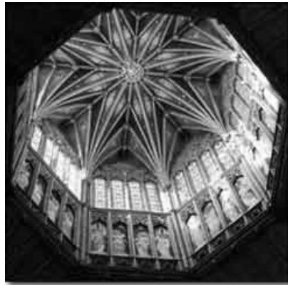
Fig.5 The famous octagon of Ely Cathedral was seriously damaged by the deathwatch beetle
