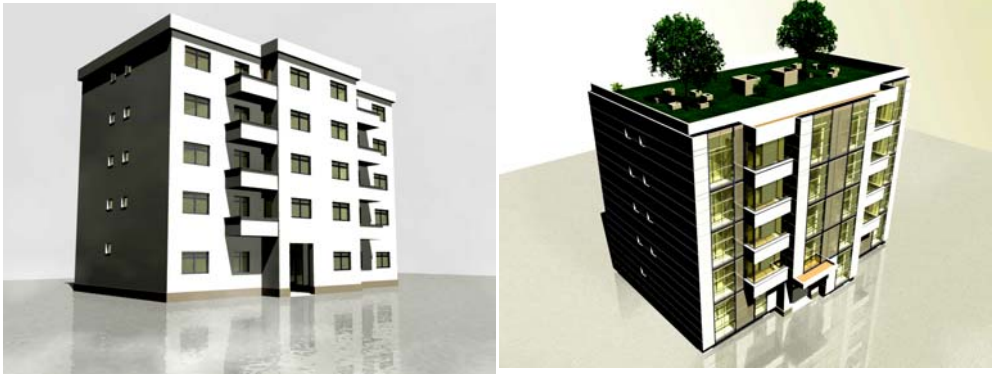
Figure 4. Existent façade versus modernized double skin facade
