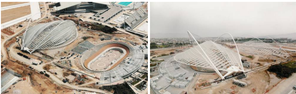
Figures 20 and 21. The roof of Velodrome before and after sliding
