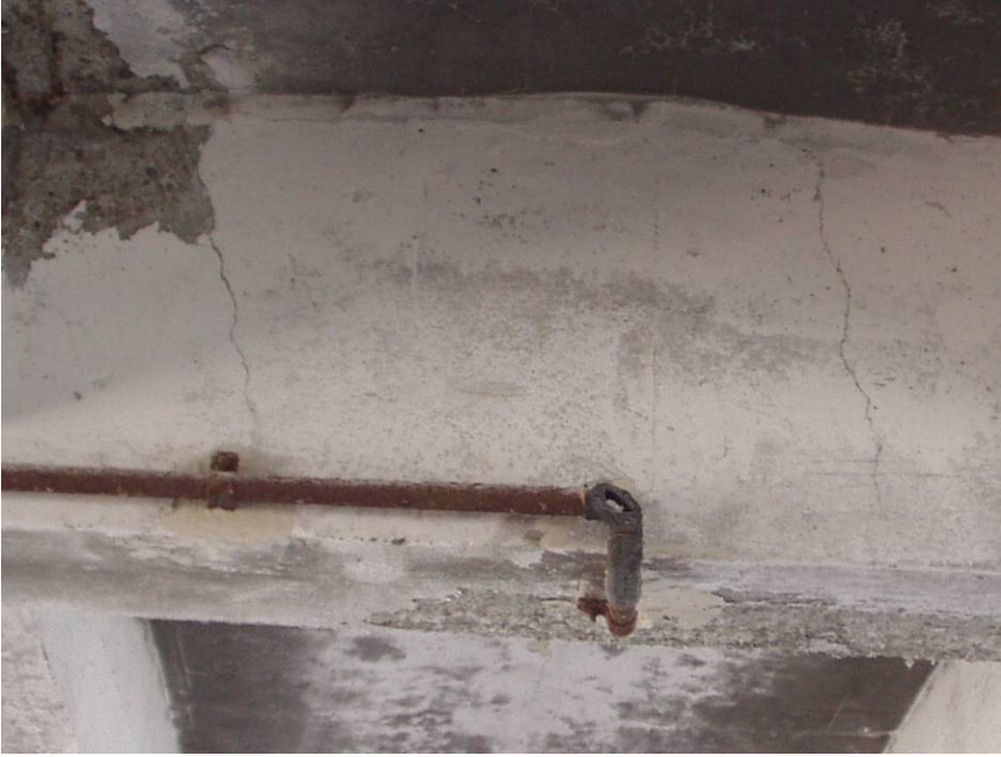
Figure 3. Cracks on transversal girders
