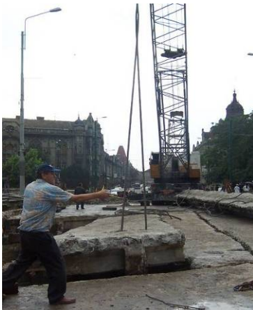
Figure 8. Demounting of the initial central bridge deck
