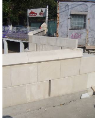
Figure 12. The new chalkstone parapet
