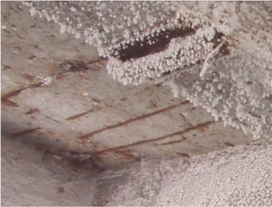
Figure 5. Degradation of the floors
