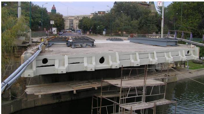
Figure 10. The short cantilivers were repaired, protected and consolidated
