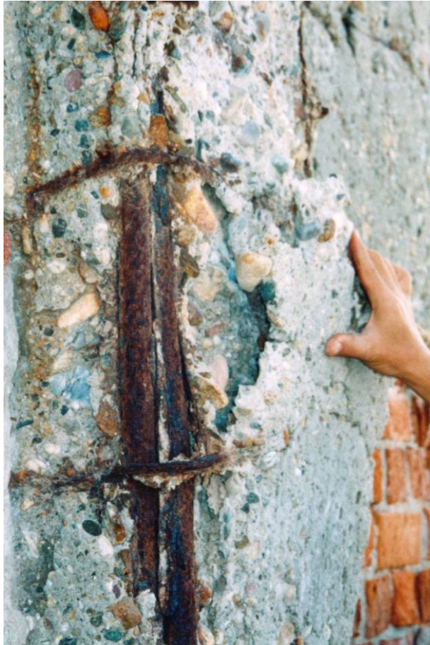
Figure 2. Degradated column
