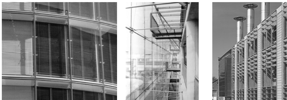
Figure 11, 12, 13: Double glazed ventilated facade (RWE Headquarters by Ingenhoven, Overdiek, Kahlen and Partners); sun space in the form of double glazed facade (Thomson Advertising Agency by Schneider&Schumacher); solar chimneys and sun shade (BRE Office of the Future by Fellden Clegg Architects)
