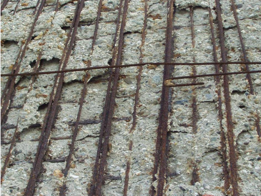
Figure 4. Degradation of the walls silo
