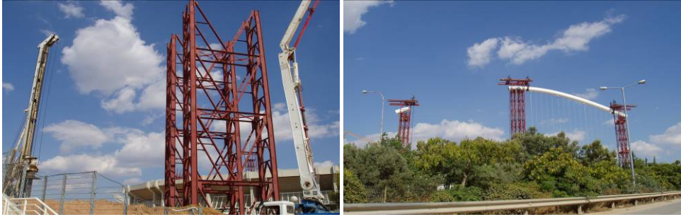
Figures 7 and 8. The temporary towers and the erection of the arches
