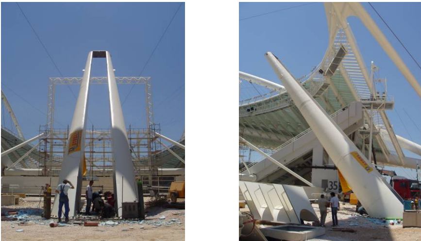
Figures 38 and 39. The Torch during erection
